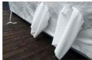
Air Conditioning Vents
